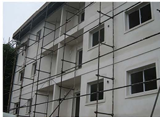
IMPLEMENTED FACE OF SOUTH FACADE
