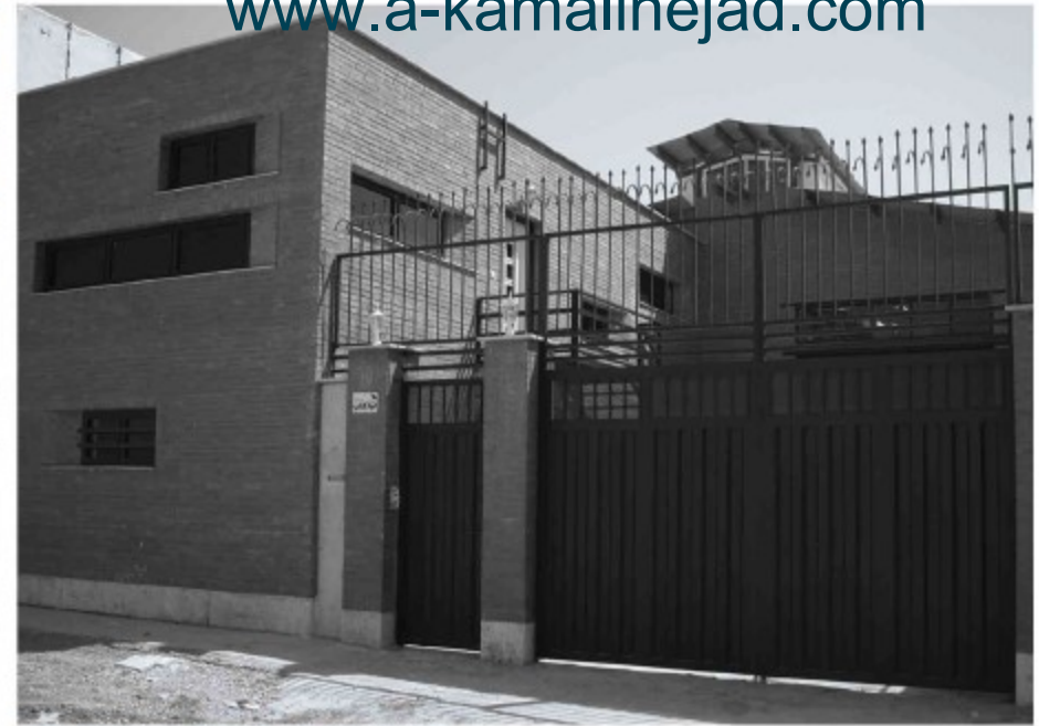
IMPLEMENTED FACE OF NORTH AND WEST FACADES
